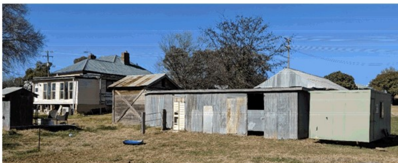
View from the rear showing the form of the Stable
