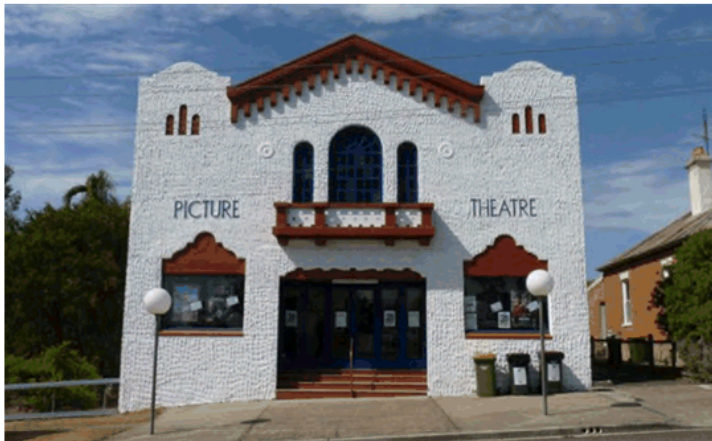
The cinema at Dungog in the same style, noting the simple white and terra-cotta colours plus the feature Blue windows & doors
