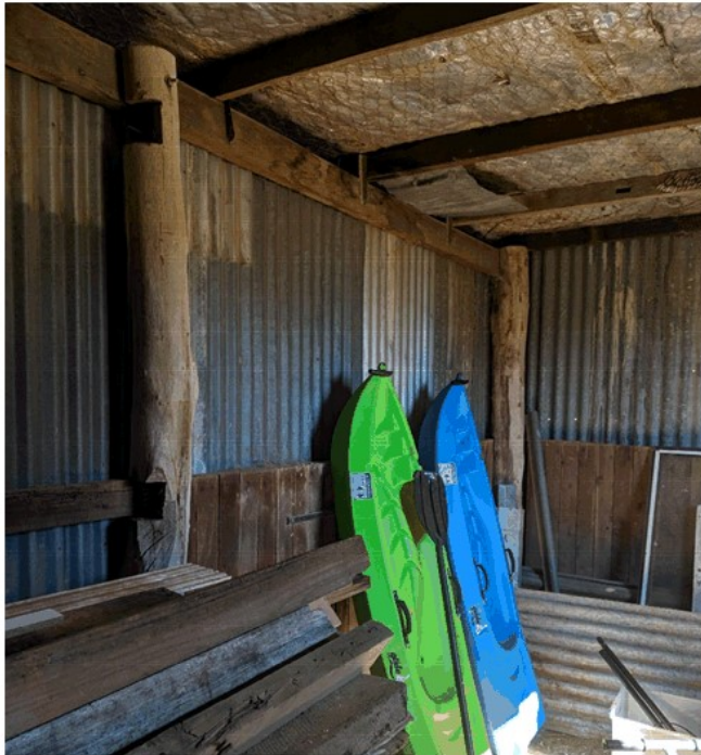
Great original posts with later roof joists
