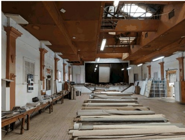
The general character of the former 600 seat Cinema space
