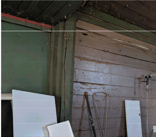
Original timber to be retained.
