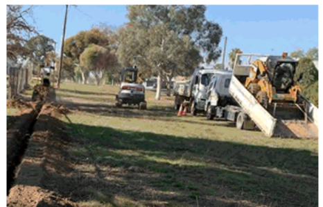
Manildra Water Infrastructure Works
