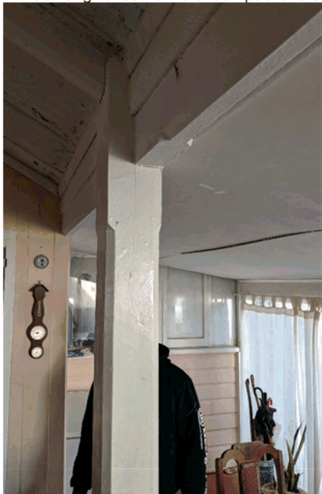
4. An original verandah post to be retained and re-used
