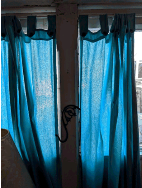
1. Original timber post with chamfers and similar chamfered lintel beam for reuse.
