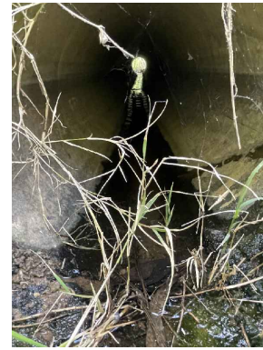
VIEW FROM DOWNSTREAM
