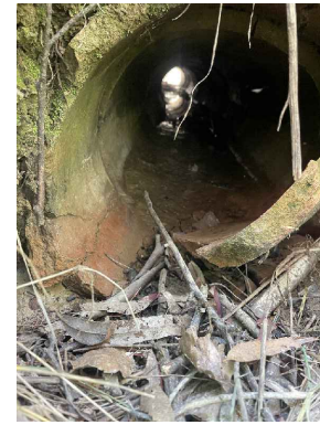
VIEW FROM DOWNSTREAM
