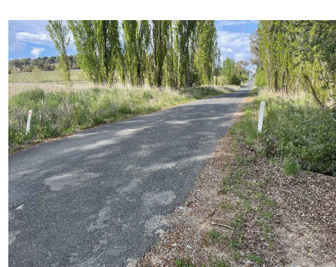
LOOKING SOUTH AT CULVERT 1
