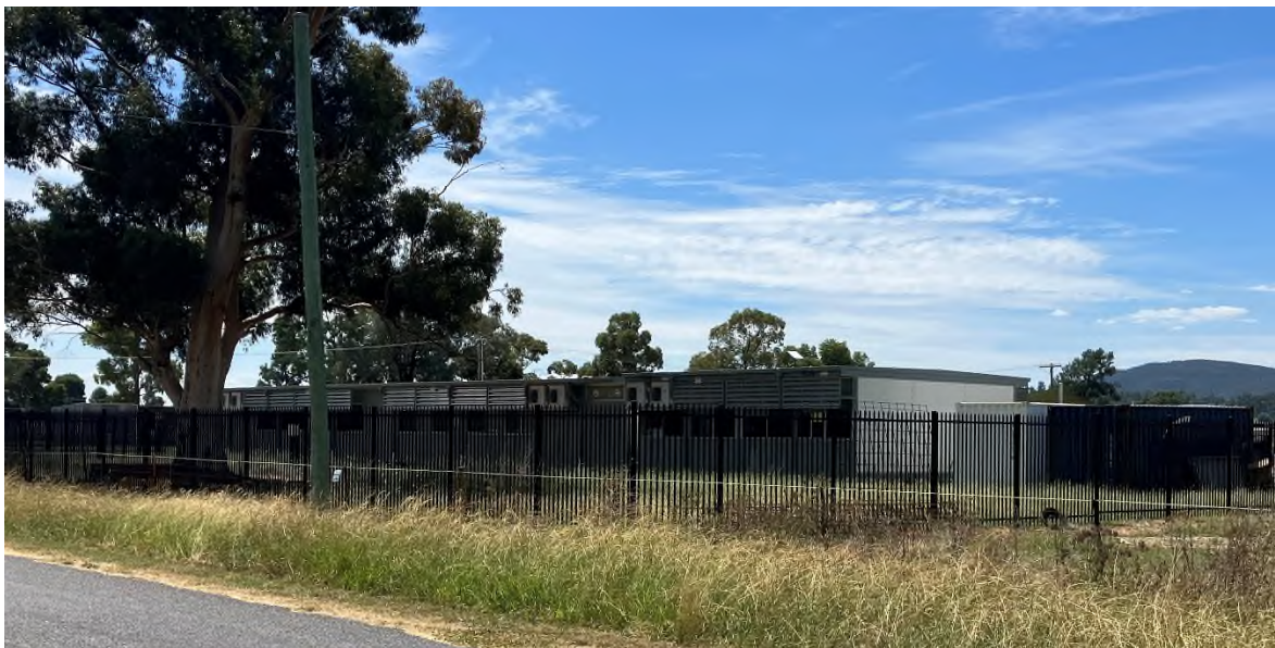
Figure 5: Temporary site of pre school – Noble Street, Eugowra
