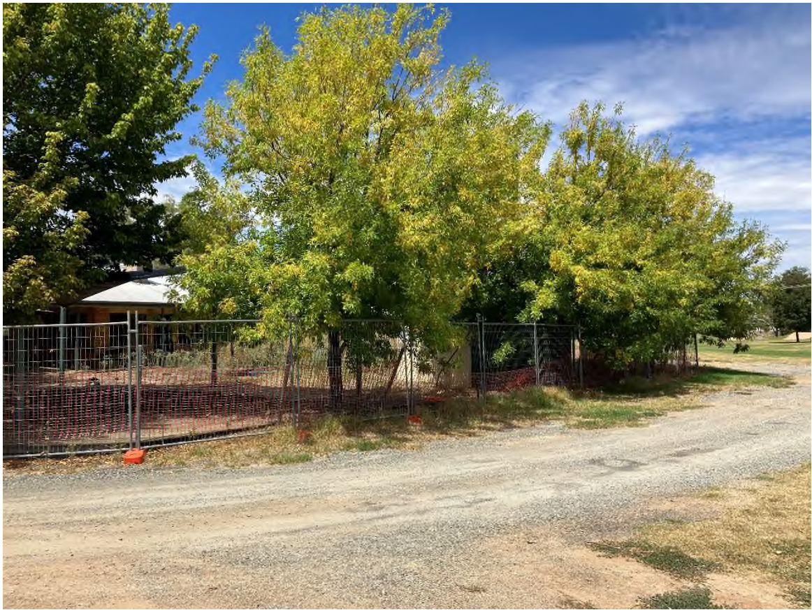
Figure 4: Flood damaged former pre school site – Nanima St, Eugowra
