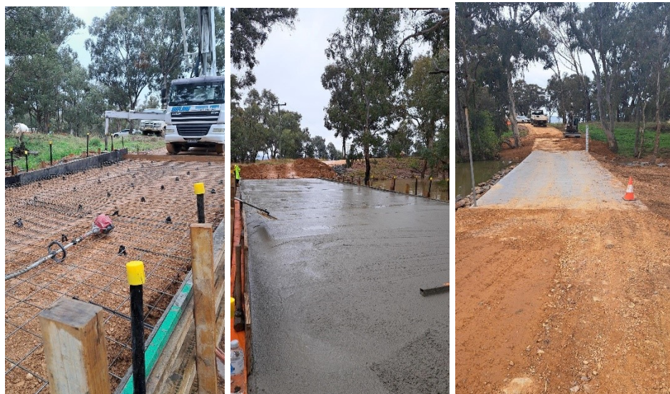
New concrete causeway for Nyrang Creek crossing on Nangar Road
