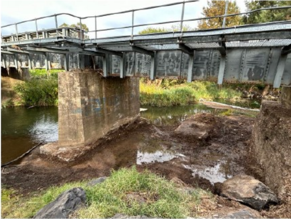
Rail Bridge 1 in Molong following debris removal
