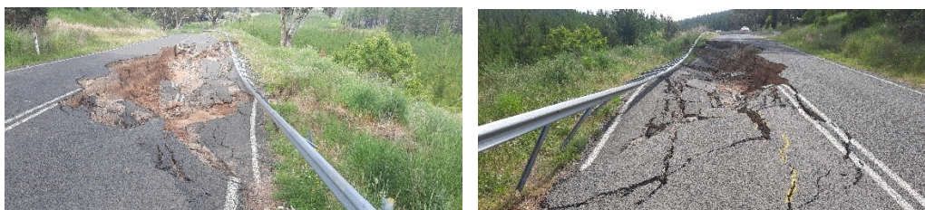
Four Mile Creek Road – 01 December 2022
