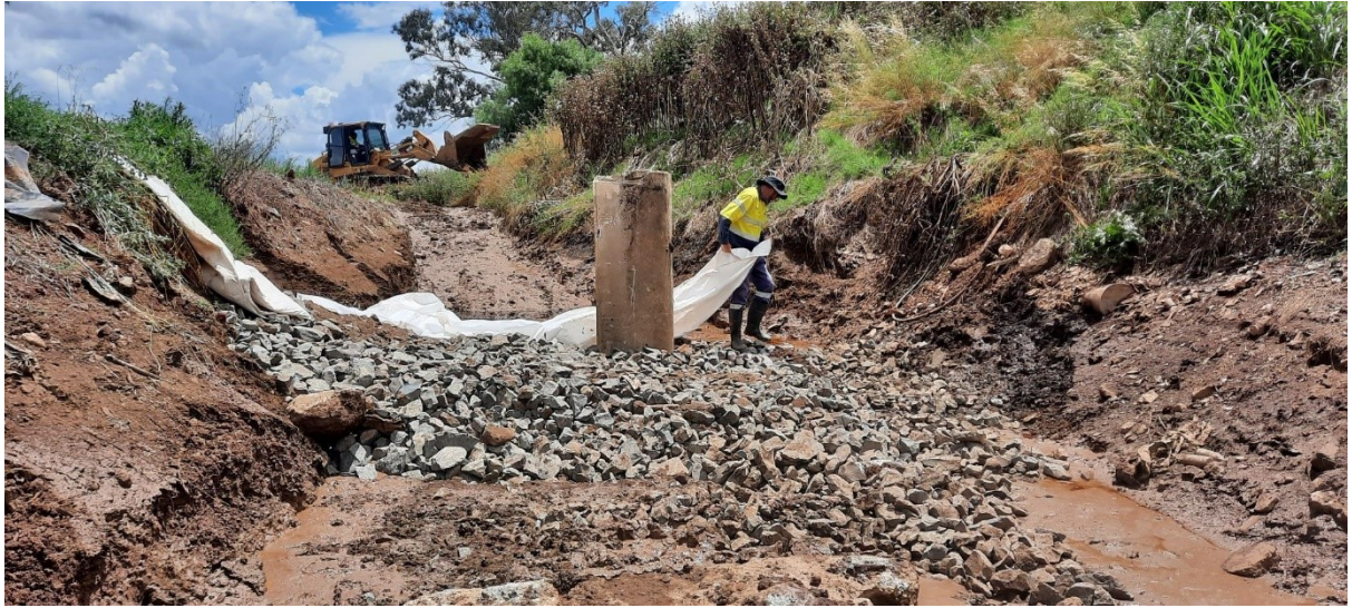
Coverage of ballast rock with membrane
