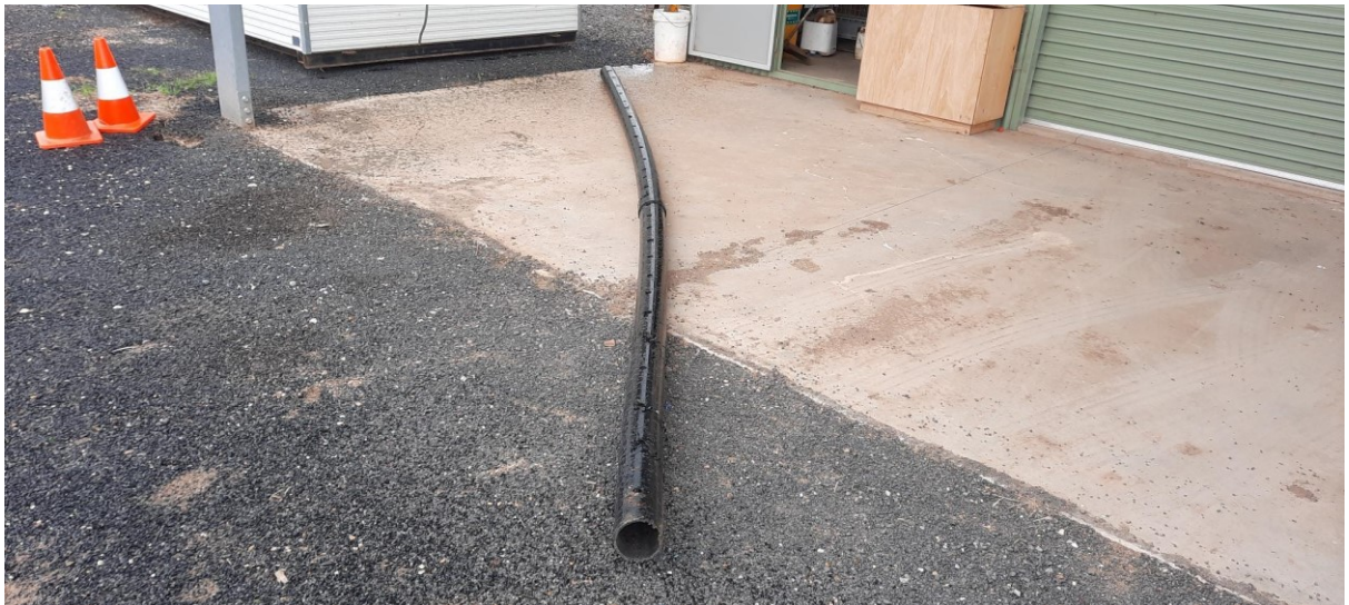
Recyclable pipe from tip used for drain line
