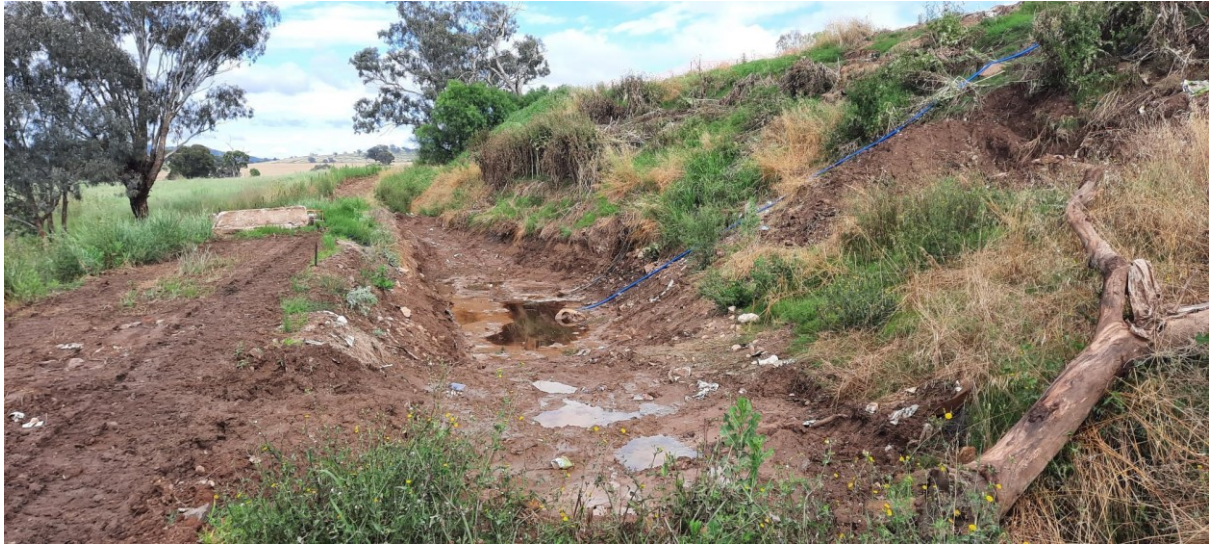
Pit empty ready for concrete pad, ballast
