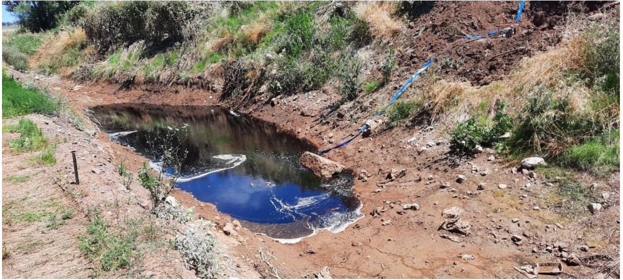
Draining of leachate pit, this took over 8 days to empty at a depth of over 3 mtrs in the centre
