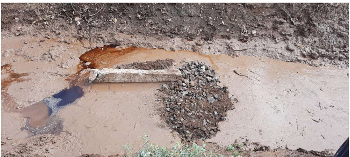
Recyclable pipe from tip used for drain line
