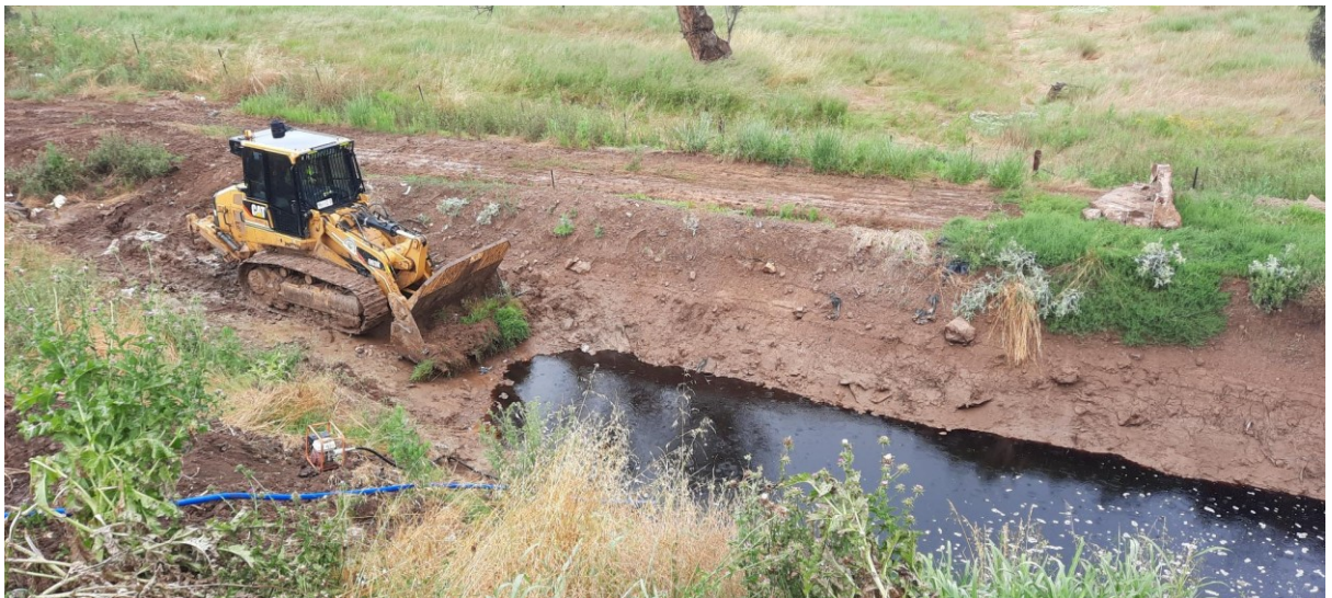
Draining of leachate pit, this took over 8 days to empty at a depth of over 3 mtrs in the centre
