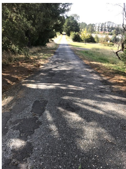
Existing single lane road surface 4m wide
