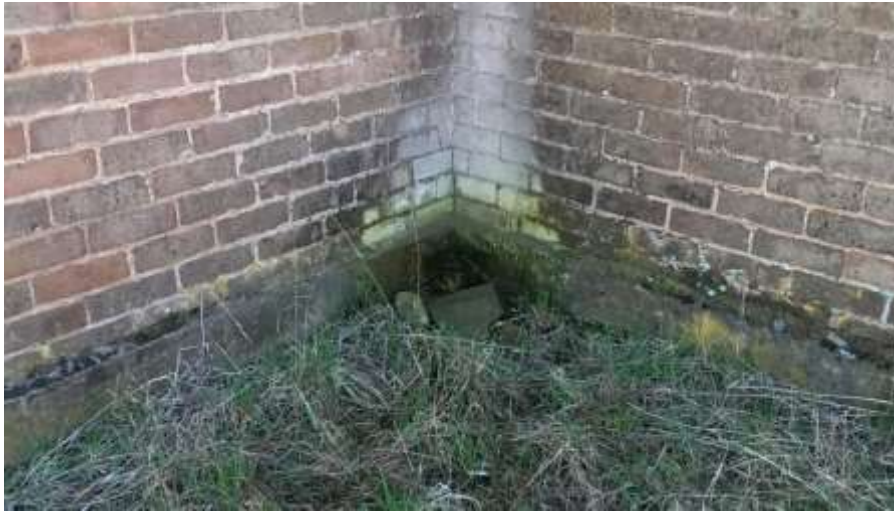
Figure 8 The solution is an extra downpipe in this area with the water carried 4m clear.
