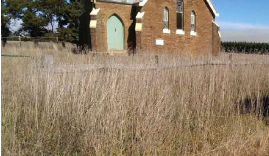
Figure 1 General view of roadside. Council will endeavour to increase the mown verge from the corner evident in the following image.
