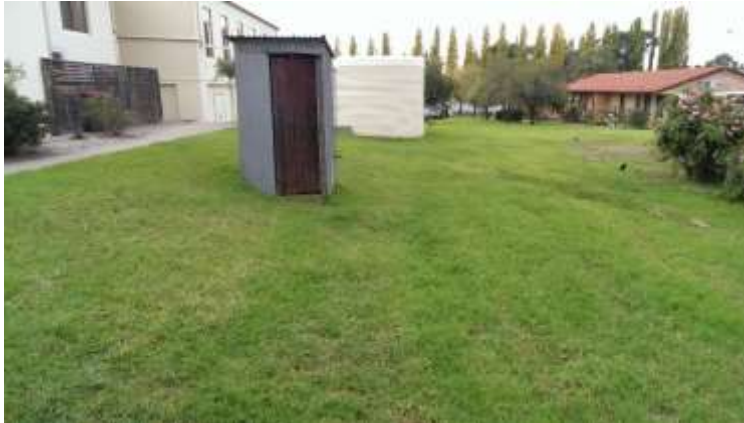
Red paint to toilet door
