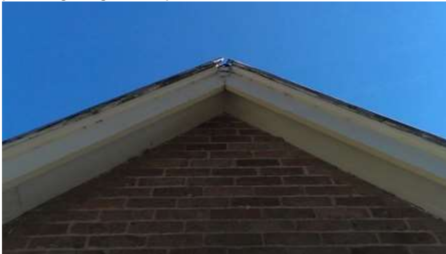
Figure 5 The missing cross leaves the two barge roll flashings open and water can affect the roof and barge boards
