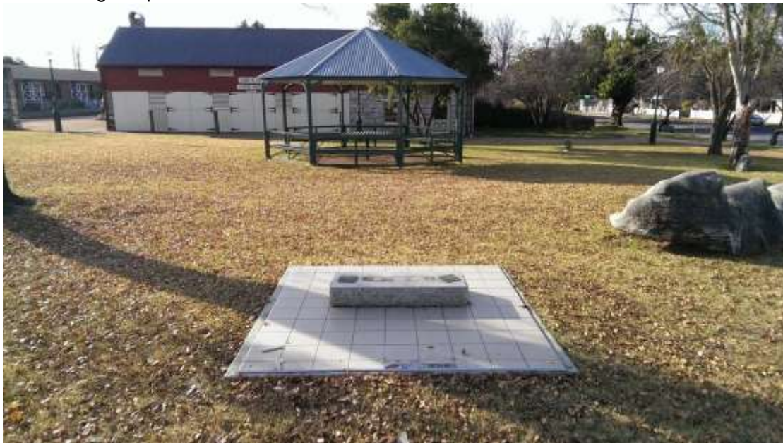
A view from Bank Street looking towards the rotunda structure with the rocks to the right and the tiled concrete slab in the foreground.
