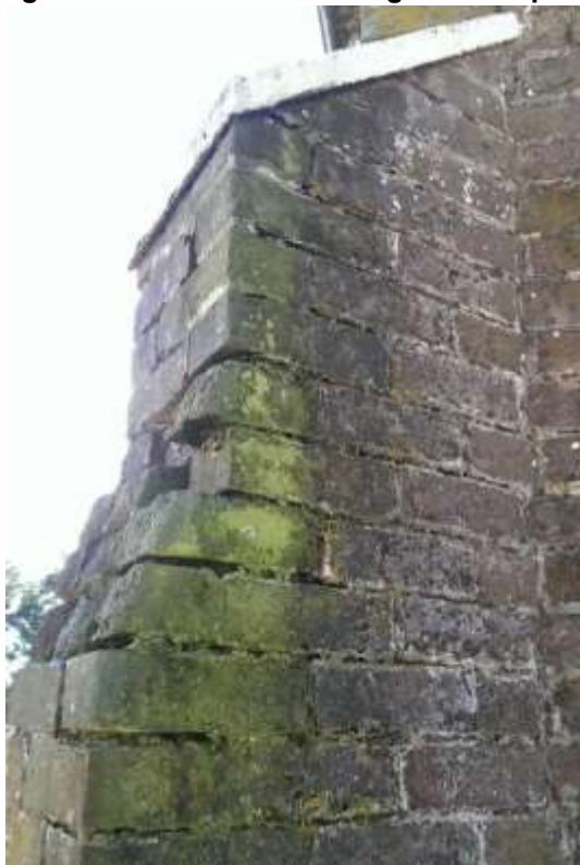
Figure 14 Water damage
