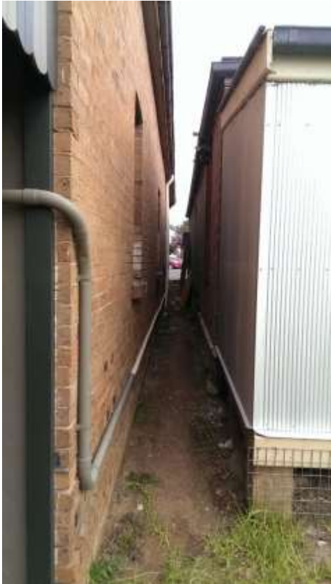
View of the side passage between the two buildings.
