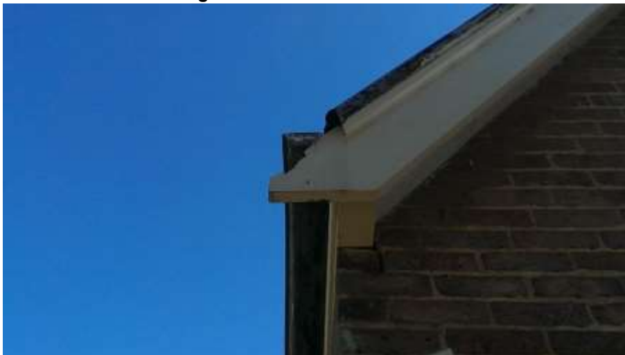
Figure 5 The missing cross leaves the two barge roll flashings open and water can affect the roof and barge boards
