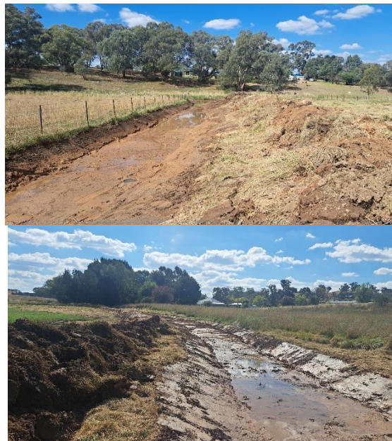
Merga Street drainage
