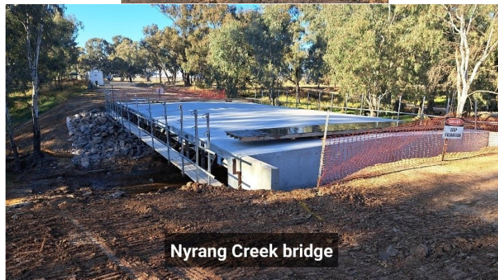
Nyrang Creek Bridge
