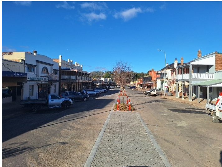
Molong Main Street – Completed Hotmix repairs
