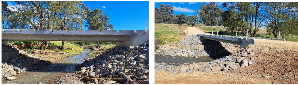
Completed work at Canomodine Lane Bridge
