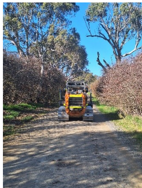
RERRF Work being undertaken on Favell Road
