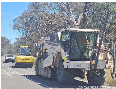
Work underway on Renshaw McGirr Way
