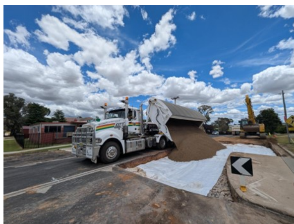
Side Tipper unloading road base to dig out on Wellington Street
