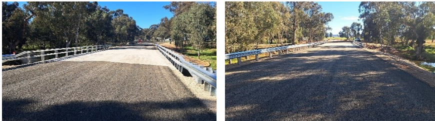
Completed work at Nyrang Creek Bridge
