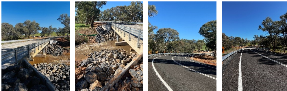
Completed Work at Washpen Creek Bridge
