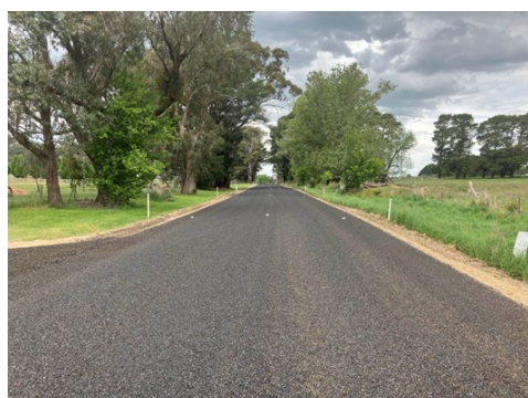
Works on Four Mile Creek after sealing.
