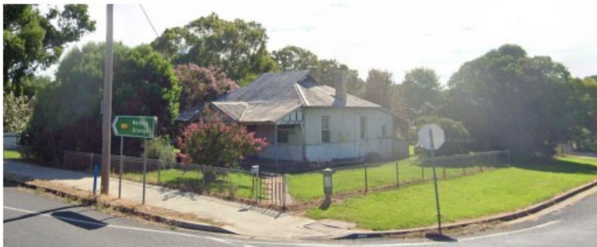
Figure 1 Existing dwelling to be demolished
