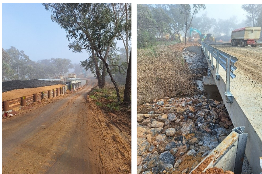
Washpen Creek Bridge – 24 July 2024
