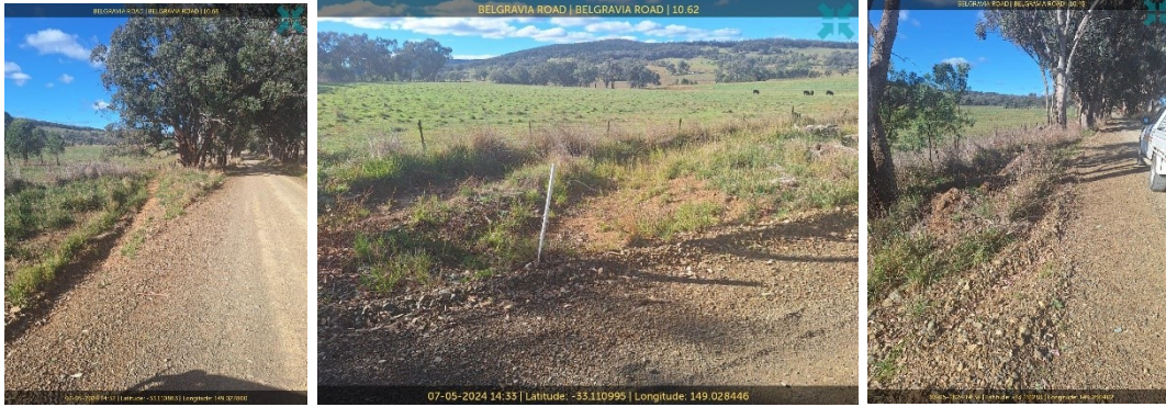
Belgravia Road – Before Drainage work
